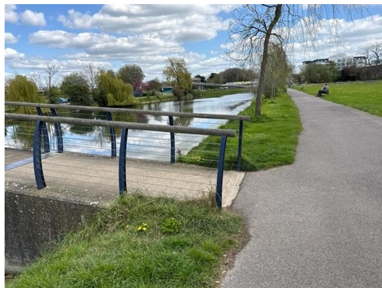
Photograph 2 : Bridge Across Waterbody
